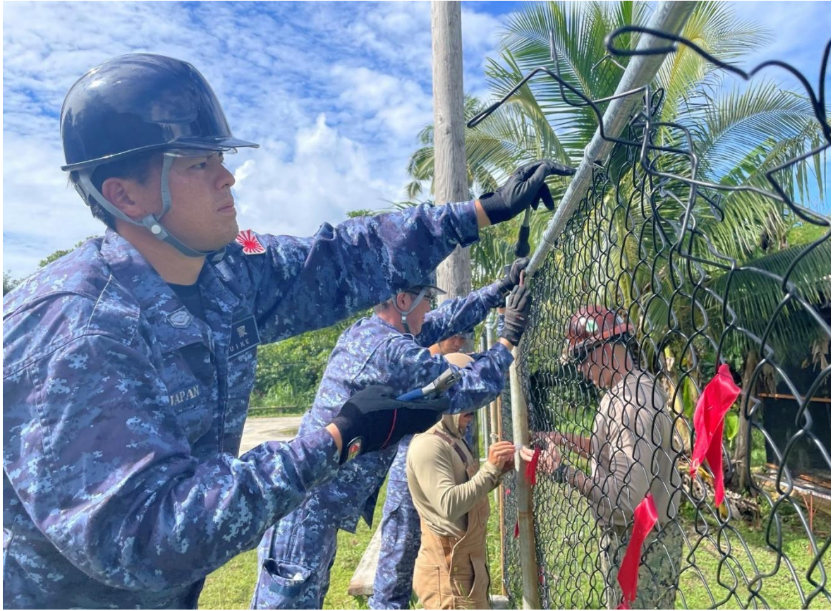
Facility repair training
