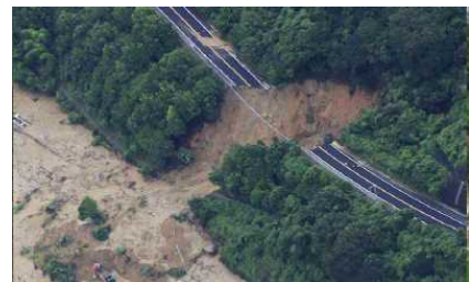
Roads cut off by sediment
