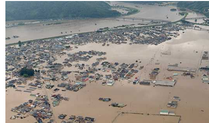
Flooding in large residential areas
