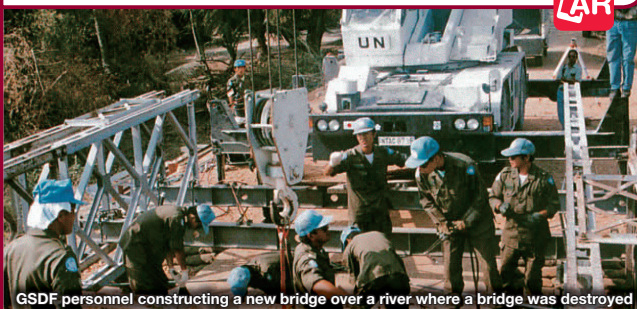
GSDF personnel constructing a new bridge over a river where a bridge was destroyed
