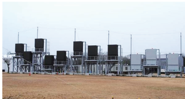
The next generation warning and control radar units at the time of technical demonstration
