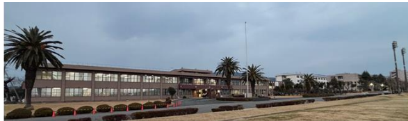
Renewal of aging facilities (image)
