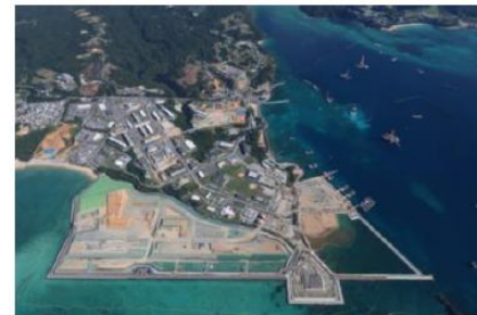
Construction of the Futenma Replacement Facility
