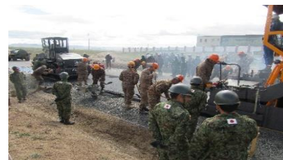
Field Training in the PKO (facility) field
