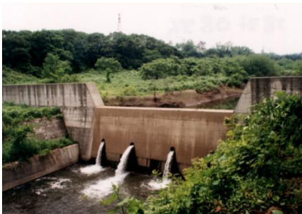
Sand Control Dam
