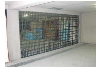
Reinforcement of Building Structure through External Reinforcement and Construction of Additional Internal Walls (conceptual image)
