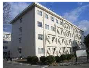
Reinforcement of Building Structure through External Reinforcement and Construction of Additional Internal Walls (conceptual image)
