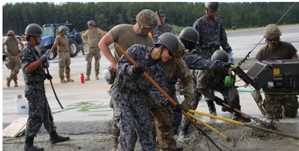
Japan-US Airfield Damage Repair Exercise
