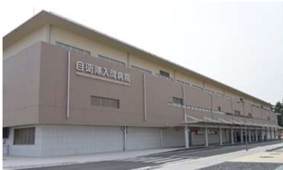
The establishment of the self-defence Force Iruma Hospital
