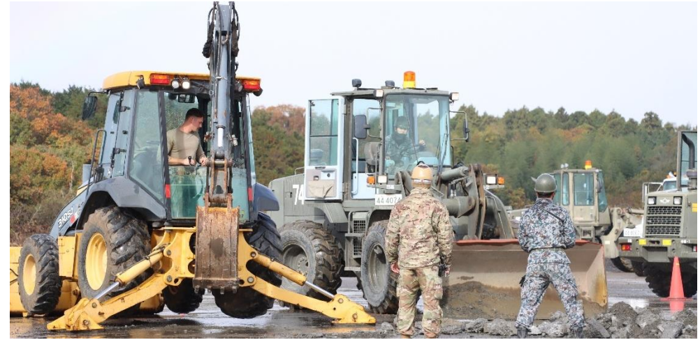
JPN-US Rapid Airfield Damage Repair Training (NOV 2024)
