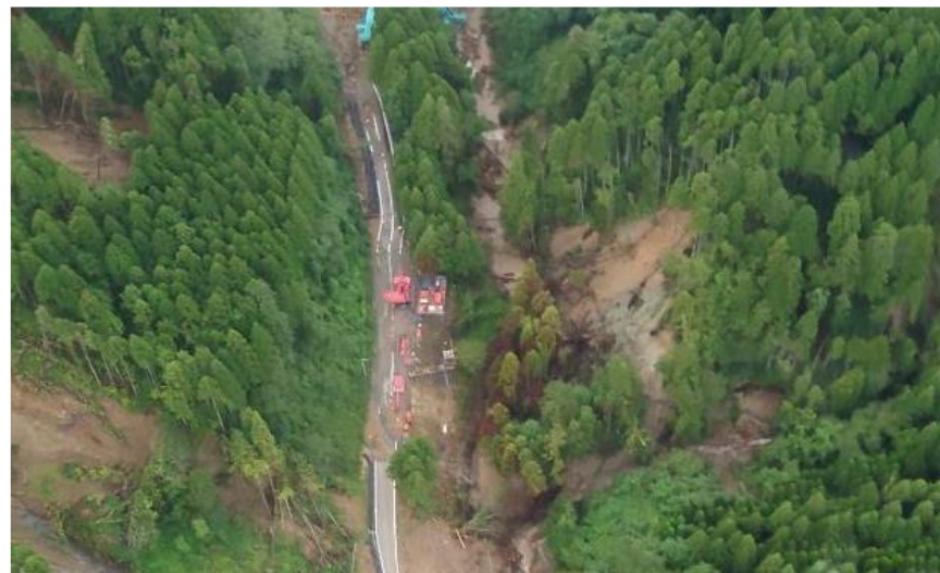
Information gathering by UH-60J (landslide) (22 SEP)
