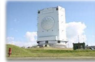
Aircraft Control and Warning Units
