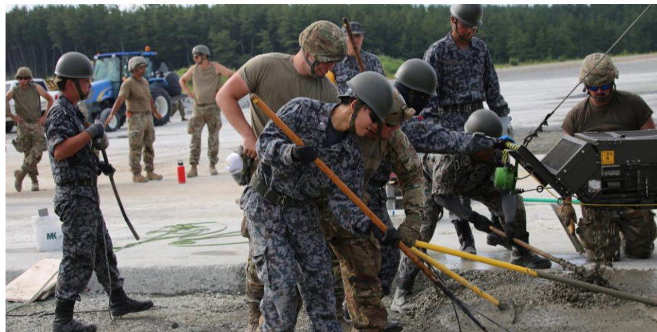
Japan-US Airfield Damage Repair Exercise
