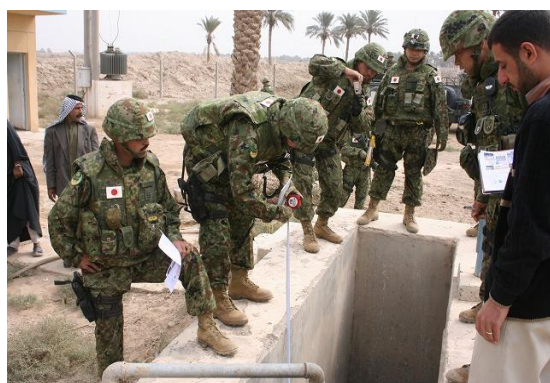
The SDF personnel to check the condition of the facilities related to the intake pump
