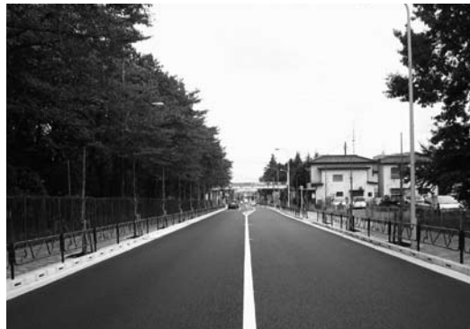
Improvements to Hamura city road route 201 were conducted as part of measures to reduce the burden of residents around the base
