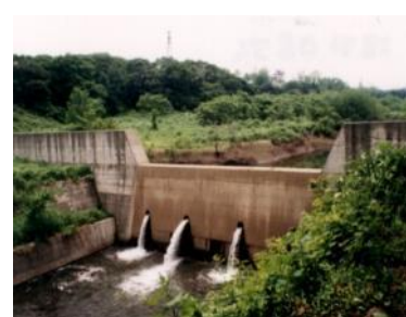
Sand control dam
