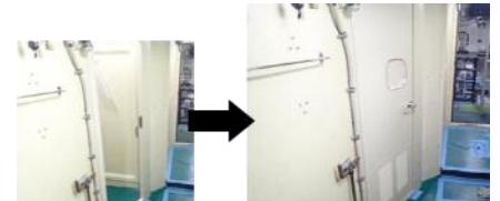
Installation of corridor doors in front of shower rooms on naval vessels
