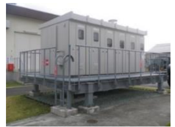
Moving electrical substations to higher ground (tsunami counter measures)
