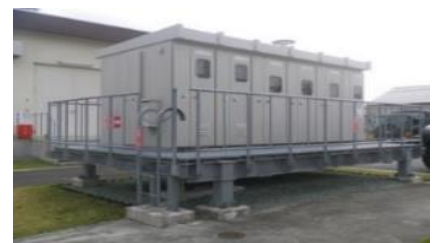
Elevation of Substation Facilities (Measures for Tsunami)
