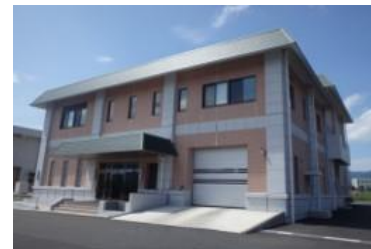
Night-Soil Treatment Plant
