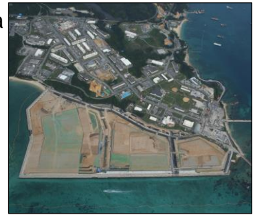
Construction of the Futenma Replacement Facility
