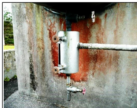
Corrosion of fuel tank for equipment facility
