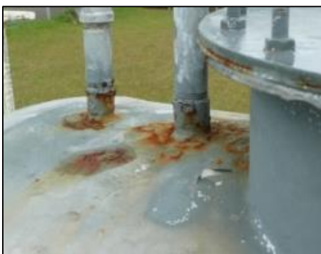
Corrosion of fuel tank for equipment facility
