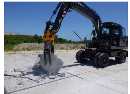
Equipment to restore damage to runways
