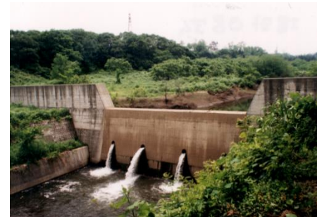
Sand control dam
