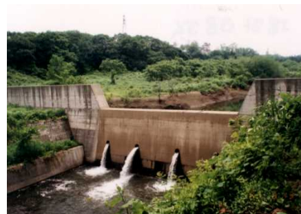
Sand control dam
