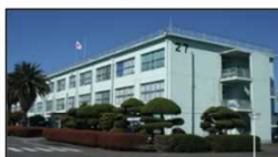
Barracks before renovation
