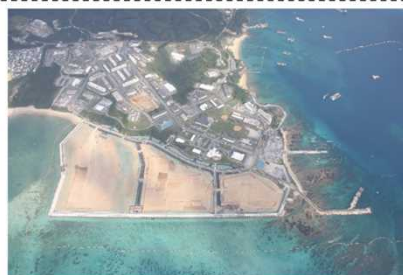
Construction of the FRF (current status)
