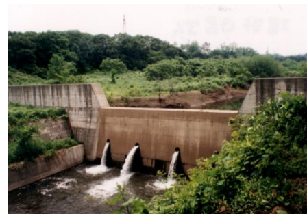
Sand Control Dam
