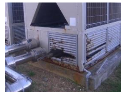
Upgrade air-conditioning facility
