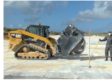
Equipment to Restore Damage in Runways
