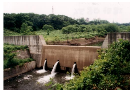
Sand Control Dam
