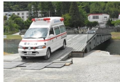
Type-07 Mobility Support Bridge (disaster management exercise)
